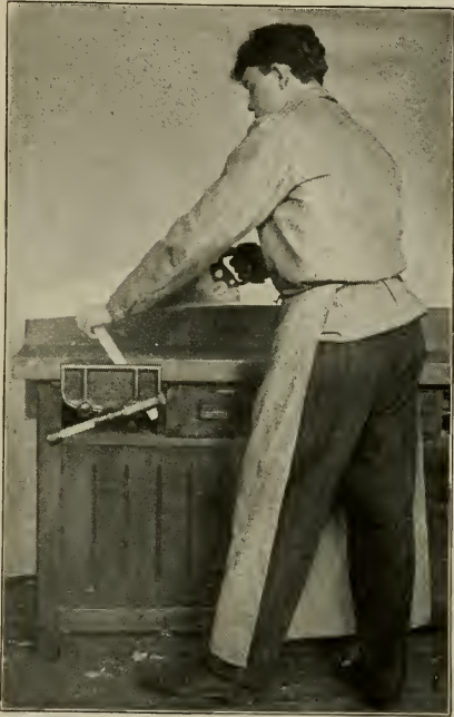
Fig. 90 - Starting Ripsaw
